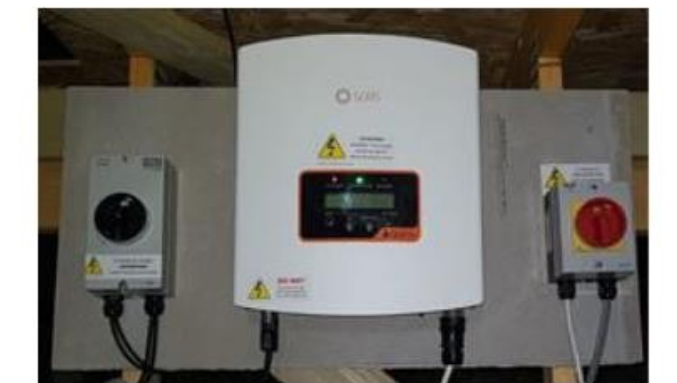
Example 2. - Inverter and isolation switches in loft space
